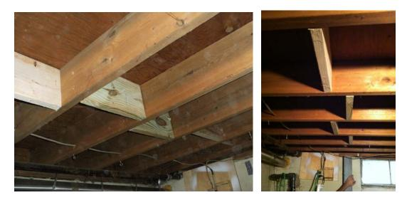
10) Once the solid blocking is in place, attach a 2"x 8"x 8' long board to the bottom of the floor joists. Bolt the 2' x 8' to the bottom of the floor joist using two 3" long by 3/8" diameter zinc-coated lag screws with washers in each floor joist. You should first tack the 2x8 to the floor joist using nails so you can drill pilot holes in the joists to prevent splitting.
