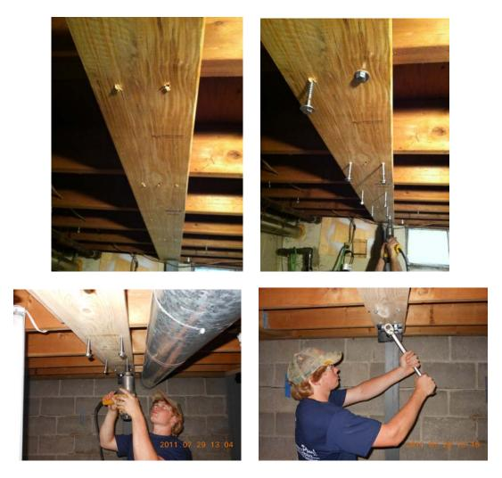
) Place the top bracket with compressed spring against the face of the beam and mark the two holes in the bracket. Remove the bracket and drill out the holes through the 2" x 8". Try to keep the holes near the center of the 2" x 8". Bolt the top bracket in place. Now follow steps 7 and 8.
