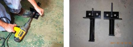
6) If the floor joists are perpendicular to the wall, secure the top of the beam using the stabilizer strap. Place the top bracket (spring Side) against the face of the beam and mark the two holes in the bracket. Remove the bracket and drill out the holes through the floor joists. Try to keep the holes near the center of the joists. Bolt the top bracket in place. **Repeat these steps for all locations before releasing the spring pressure.**
