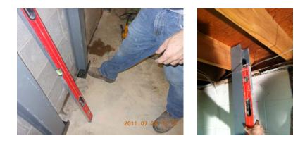
**4)** Drill holes using a 7/16" diameter drill bit (keeping the angle and beam in place to guide your locations). Drill both holes deep enough to accept the anchors. Next, use a  $\frac{3}{4}$ "socket to secure the  $\frac{1}{2}$ " x 5" anchors into the holes.
