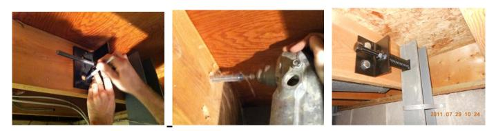
7) Carefully remove the compression bolt by holding the all-thread with a pair of vise grips and turning the nut. This will prevent the all-thread from backing out of the assembly nut. The tension can be slowly applied to the beam by loosening the nut. Start in the middle of the wall and work to the ends rotating back and forth from one beam to the other. Once the nut has been completely loosened, remove the all-thread from the bracket.
