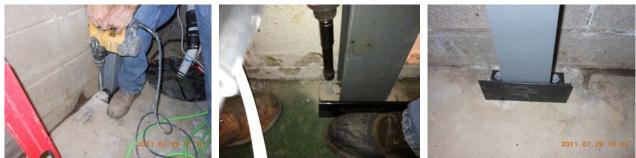
**5**) Compress the spring using the all-thread and nut. A deep socket can be used with a drill to quickly compress the spring.
