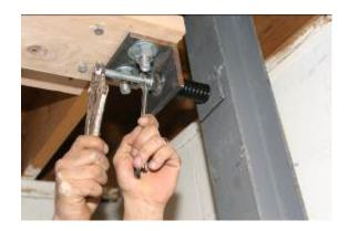
8) Install the <sup>3</sup>/<sub>4</sub>" seating bolt and tighten it using a torque wrench set at 40 pounds. Again start at the middle and work to the ends. If the spring does not align directly with the bolt, use a small punch or screw driver and hammer to re-position the bearing plate to allow the seating bolt to cleanly pass through the spring.
